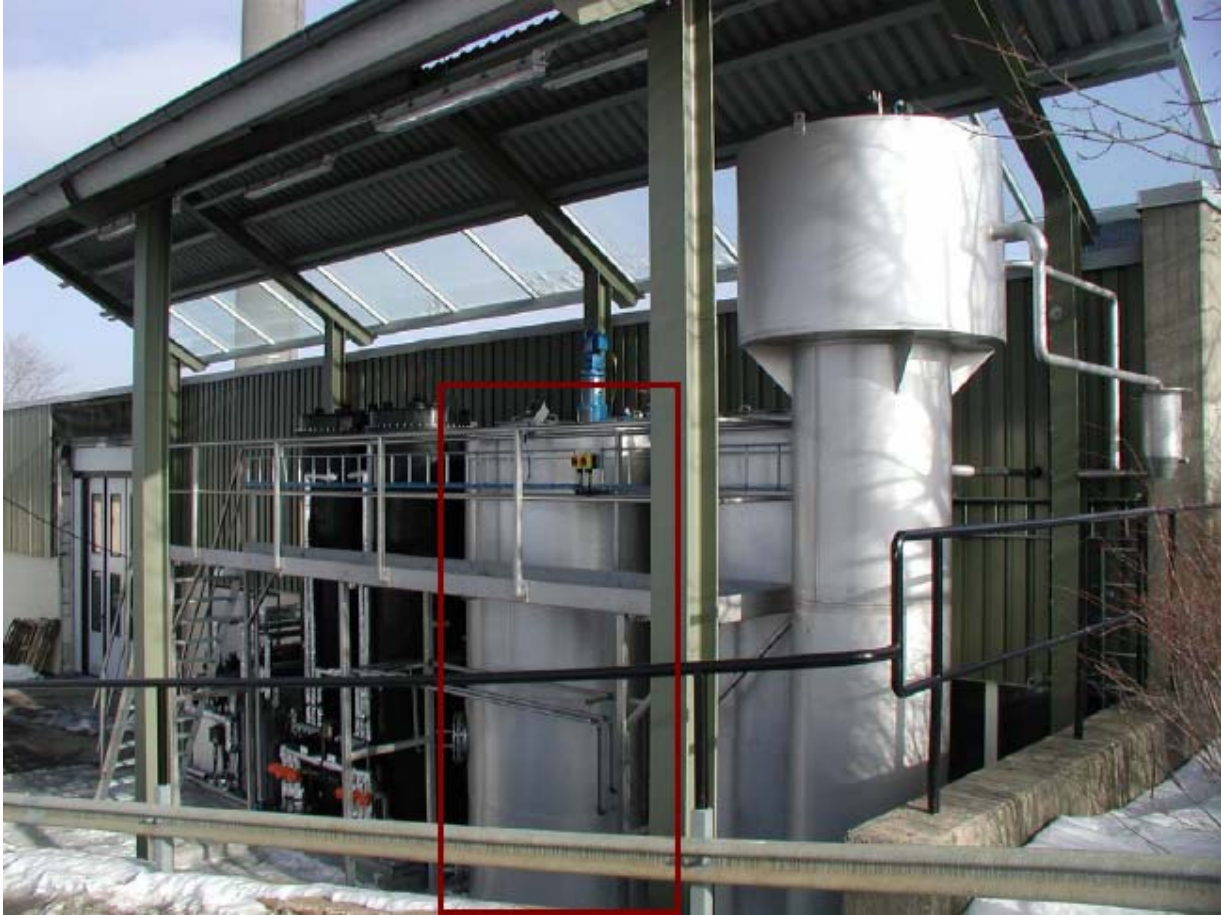
Figure 3. Anaerobic processes at Hammarby Sjöstadsvverk with the sludge digester chamber.
